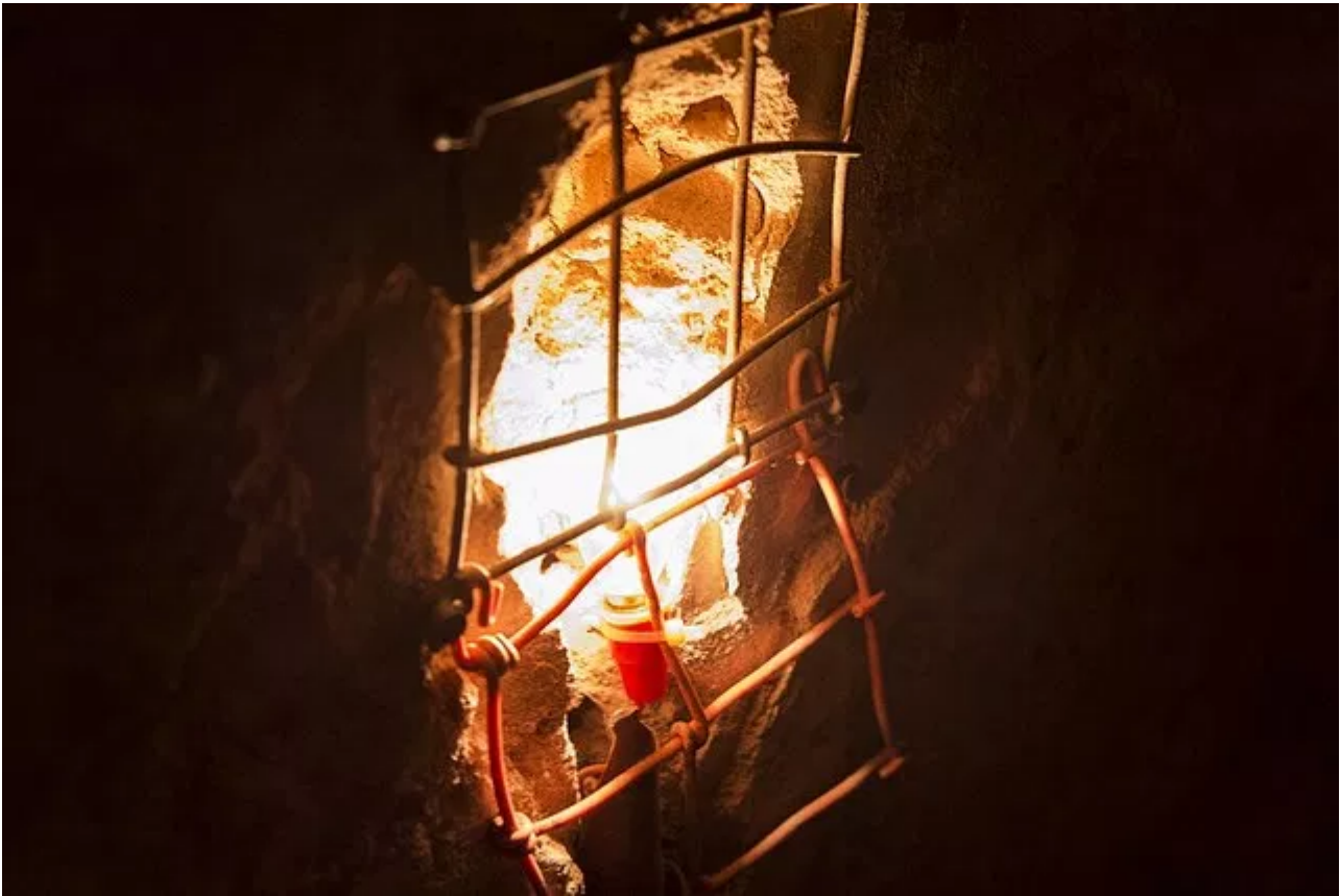
One of the many electrical lights in the tunnel, which I doubt existed in WWII
